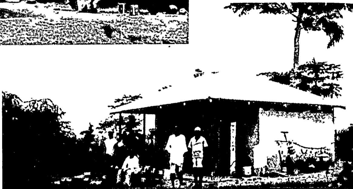
Iron-roofed Leper Building at Camp of Hope, Ogbomosho, Nigeria, West Africa
