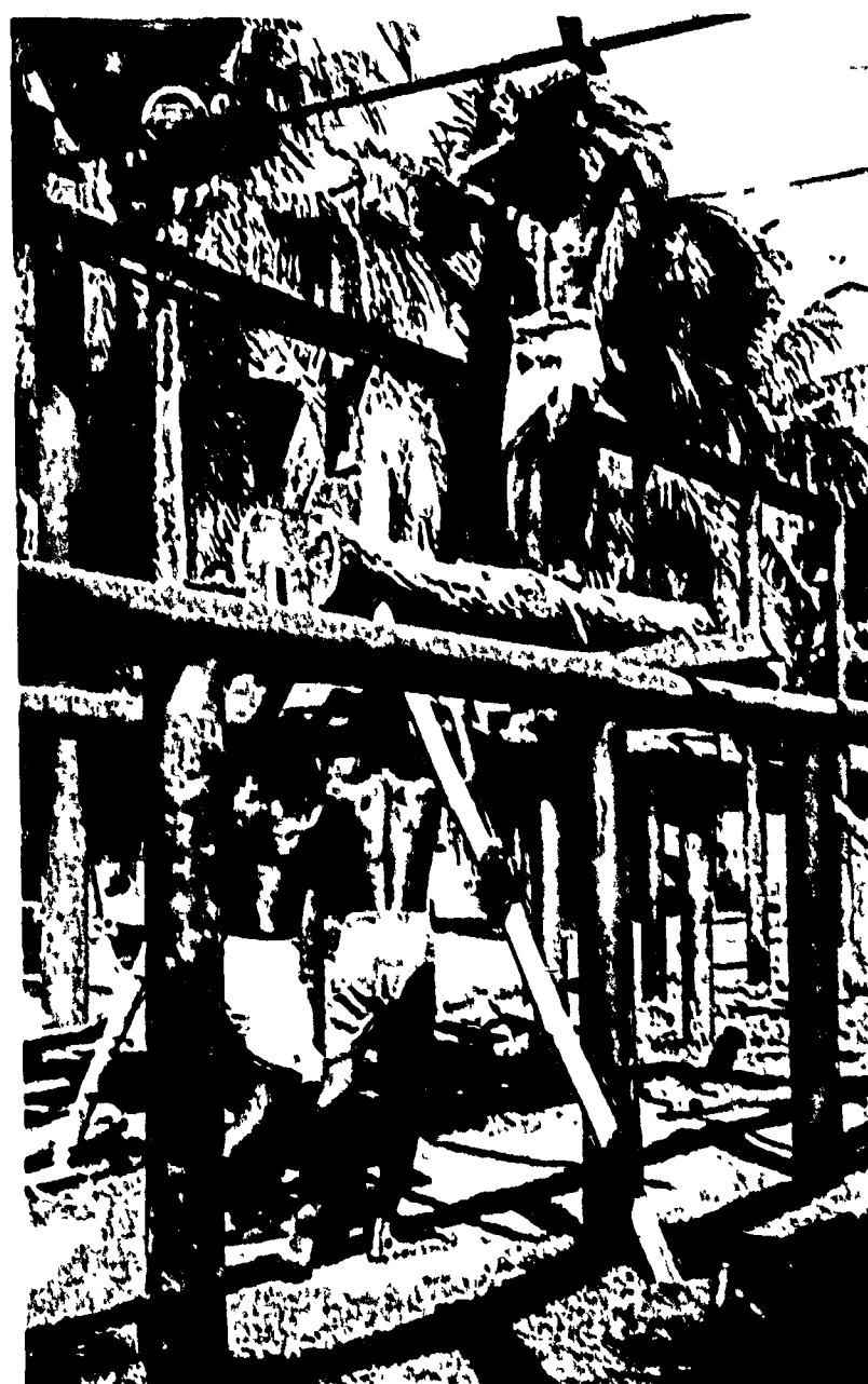
A timber supplier checks his order as a student and staff members measure delivered logs. At right, logs are sawed into planks on a gantry.
