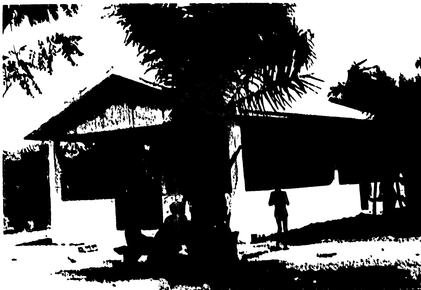
New chapel building at Klemé, Togo. Members are to complete three walls.
