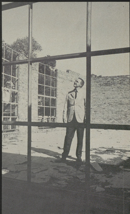
Church and chapel construction
