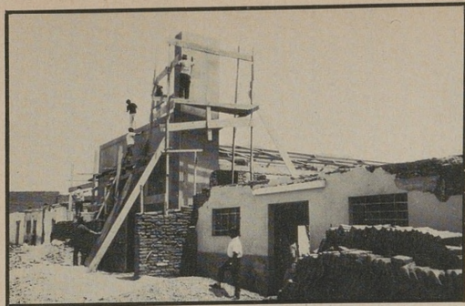
Building of brick and reinforced concrete goes up to replace the adobe structure of Esperanza Baptist Church (old walls in foreground), severely damaged by earthquake at Trujillo, Peru.
