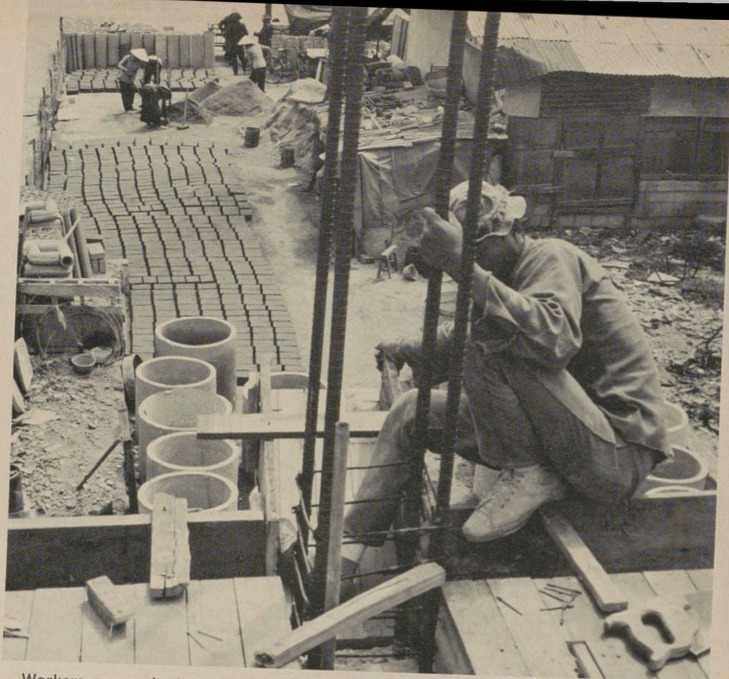
Workers proceed with construction of Baptist church building, Quinhon, Vietnam.
