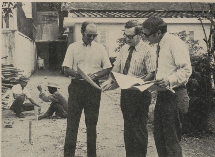
At site for new Vietnam Baptist Mission office building three Mission officers look at plans for the construction project. Left to right: Missionaries L. David Wigger, building chairman, Herman P. Hayes, treasurer, and William T. Roberson, chairman.
