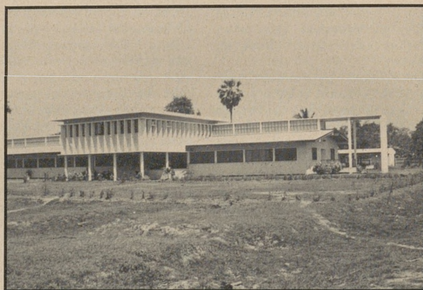
Baptist Hospital, Bangkla, Thailand.
