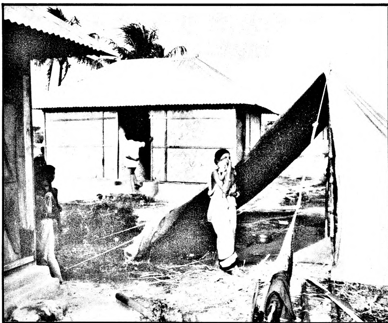
Old and new: behind temporary tent shelter can be seen a newly completed house.
