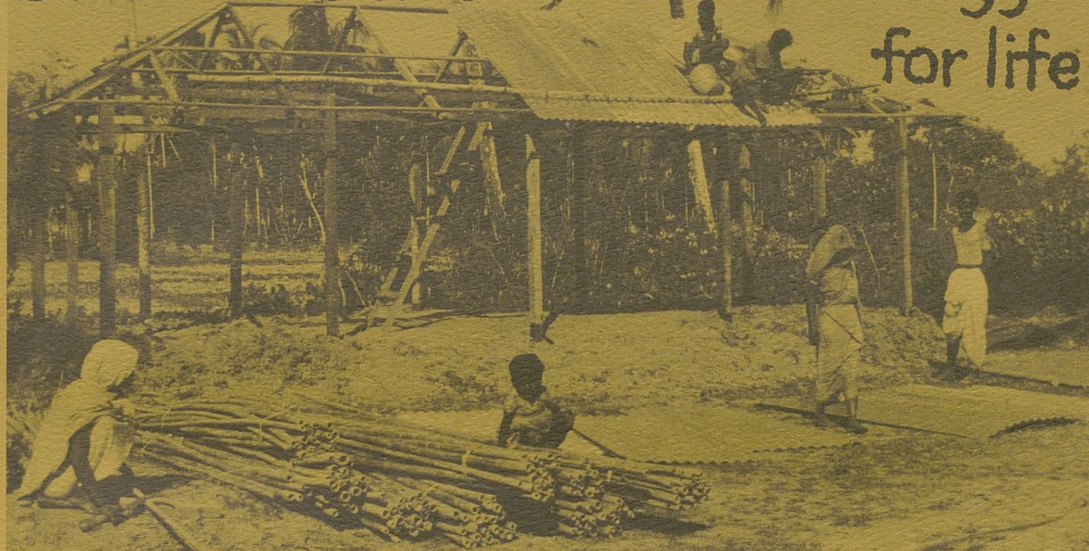
House construction project, aided by Southern Baptists
