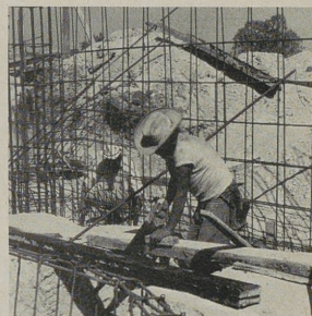
Construction has begun in Mexico City for the seminary's new home.
