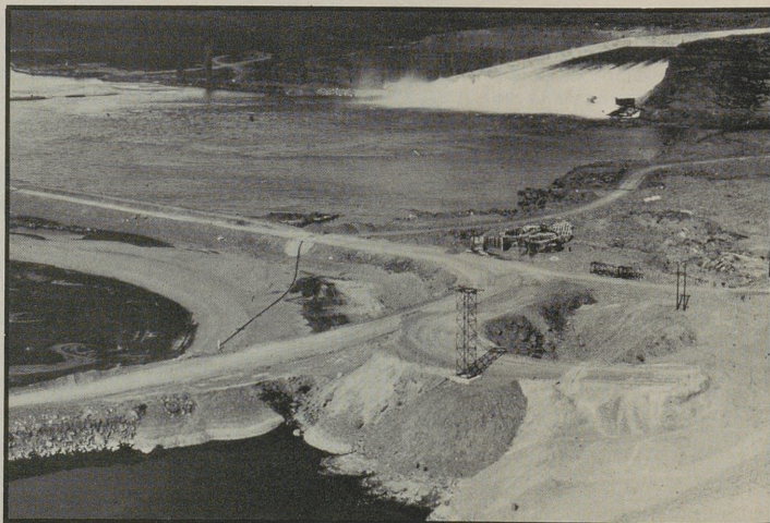
Spray rises from spillway of the dam at El Chocón.
