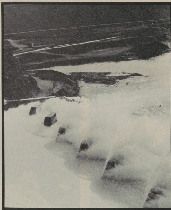
Water power is evident with only one-fourth of spillway doors open.
