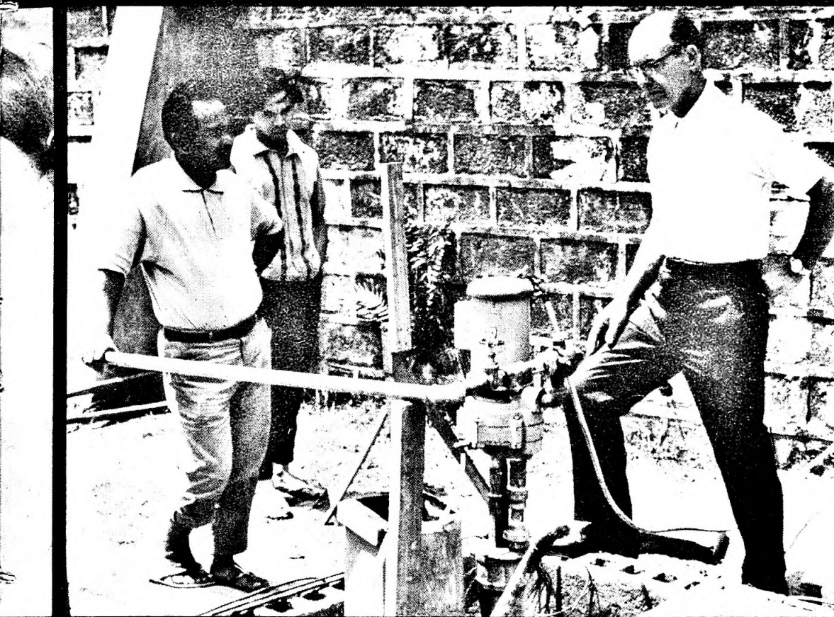
Harry Elver (r) and two workmen at the Philippine Baptist Theological Seminary and Bible School inspect newly installed pump. For his first year after retirement Elver filled in as business manager for the seminary.
