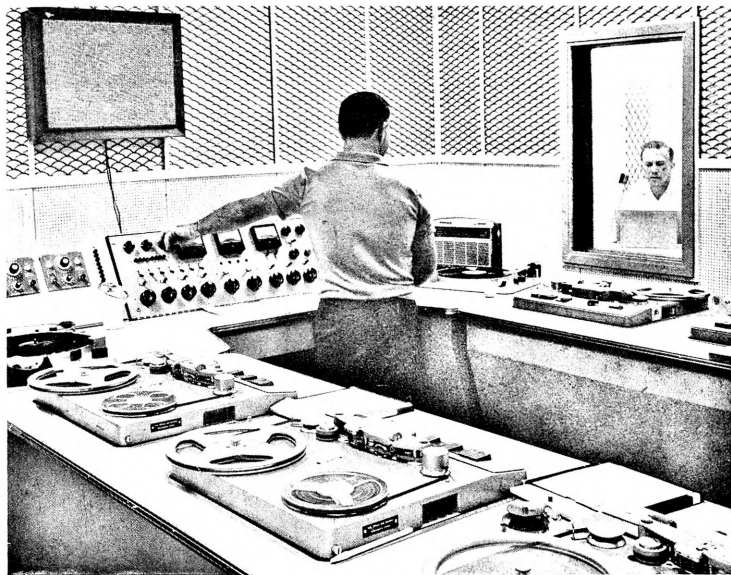
Left: One of the modern control rooms for TWR. Below: Building houses offices and studios.
