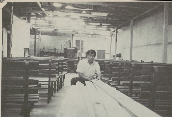
In damaged Baptist church building in Damasco, Pastor Demetrio Camay inspects lumber for repair bought with funds sent to Guatemala by the Foreign Mission Board. Through the Board's March meeting, relief funds appropriated for use in Guatemala totaled $397,000. Besides emergency relief, the funds are aiding reconstruction of Baptist church buildings, pastors' homes, and other homes.
