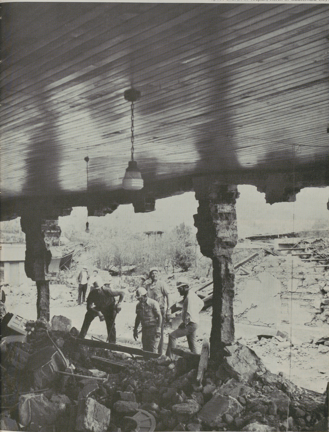
Florida laymen survey damage to buildings of First Baptist Church in Tocpan, north of Guatemala City.
