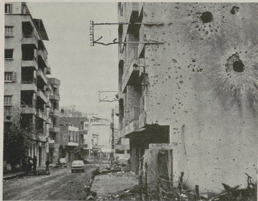
Above: Almost obscured by barbed wire, youth stands atop sandbags and surveys marks of battle. Left: Structural damage reveals ferocity and firepower of the fighting. Below: Rubble of leveled section.
