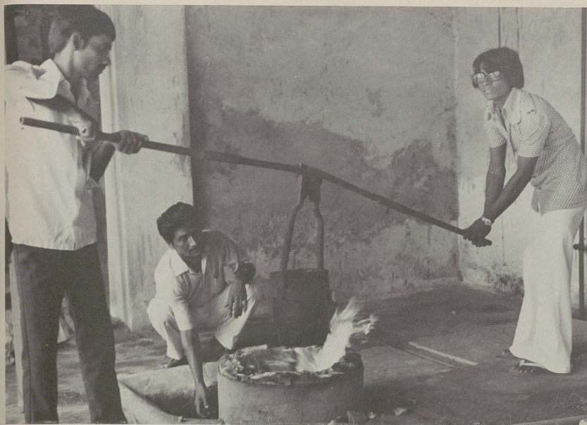
While one student tends the fire, two others carefully position container over flames in foundry.
