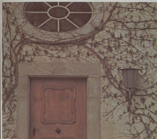
Above: Entrance to seminary campus. Left: Detail of a portion of picturesque campus building.
