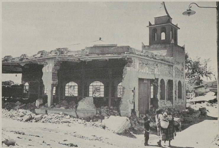
Scenes like this in Tecpán, Guatemala, greeted Baptist volunteers from the U.S. who helped in cleanup and reconstruction after the 1976 earthquake.
