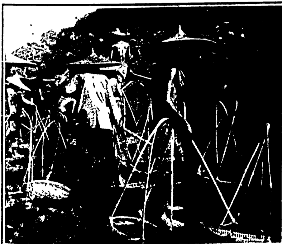
A wealthy Chinaman having given $1,000, coolies were employed and work begun on the foundations of a $100,000 hospital.
