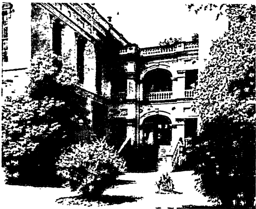
Administration Building, Baptist Bible Institute
