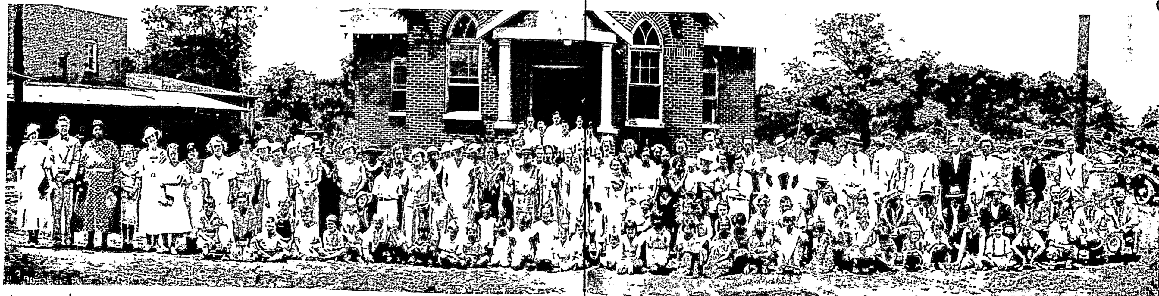
BUILDING AND CONGREGATION OF RIVERSIDE BAPTIST CHURCH, COLUMBIA, SOUTH CAROLINA This church was organized in 1912 by the South Carolina State Mission Board and has been helped by this Board nearly every year since. Now its membership totals 209, with a Sunday school enrolment of 147. Rev. J. C. Jennings is pastor
