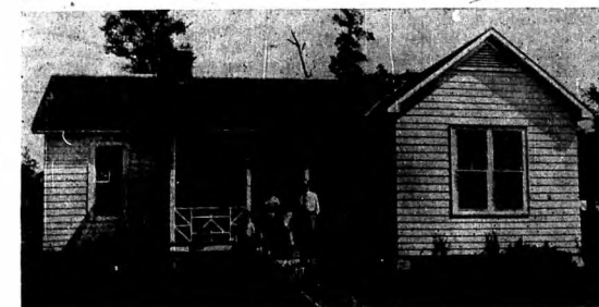
Dyess Colony Baptist Family. "Fish and Snakes Swam by the Workmen as They Felled the Trees" and Drained the Lowlands to Make Room for Modern Homes.
