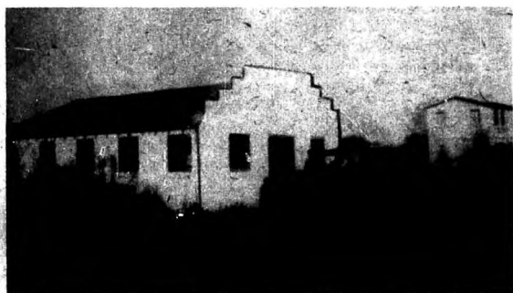
The new building of the Jerusalem Church in San Antonio. The previous owner had built it for a beer joint. It is now a house of prayer.
