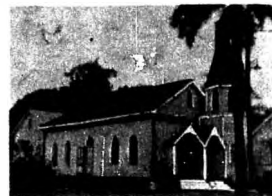
Bocas del Toro Baptist Church
