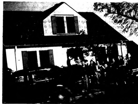
Good Will Center, Ensley, Alabama
