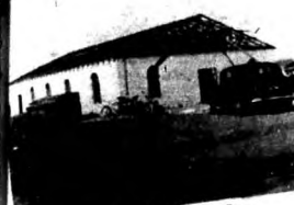
A view of the 22nd Avenue Baptist Church building, Phoenix, under construction
