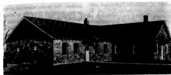
Building was constructed in units. Picture shows completed structure.
