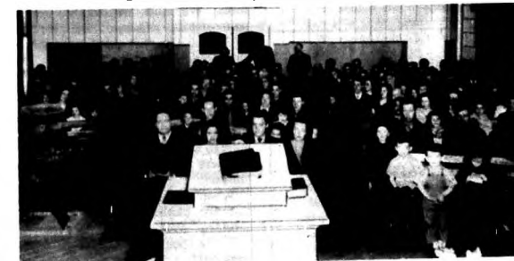
Note crude stove in First Baptist Church, Fairbanks.
