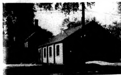
West Side Baptist Church in process of erection.
