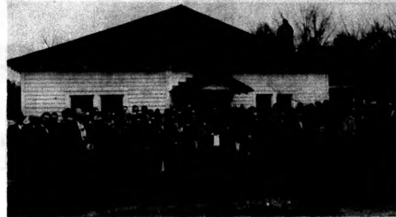
Remodeled garage serves as meetinghouse for Kentucky congregation.
