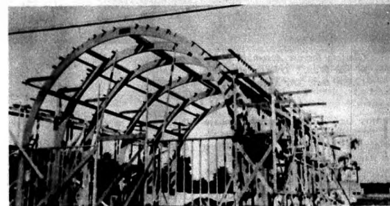
Auditorium Centinela Baptist Church under construction
