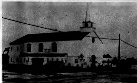
New Centinela Baptist Church building, West Los Angeles, California
