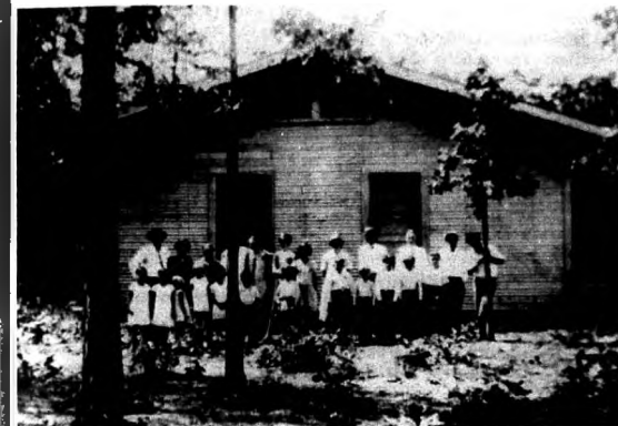
Church as it was before improvements were made.
