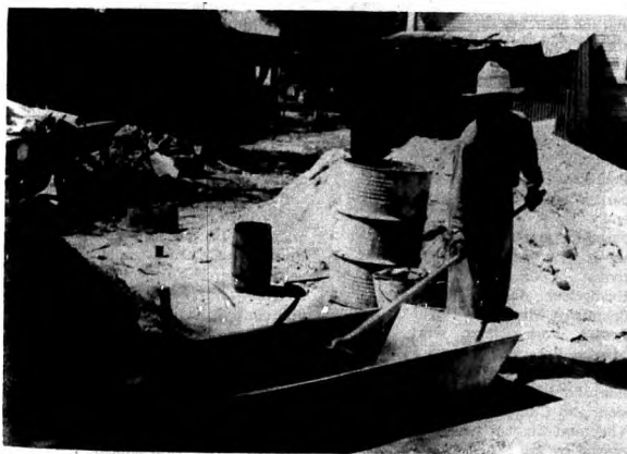
Workman mixes cement for construction job directed by Mike Cassidy.
