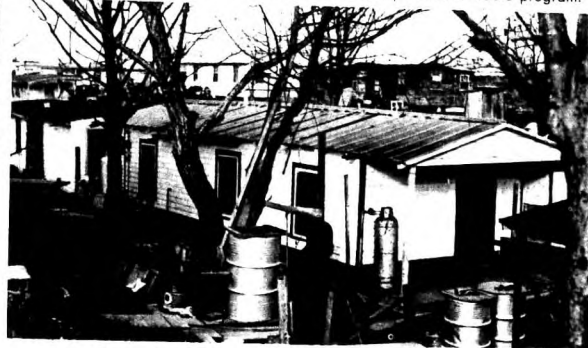
Section known as "the Pit," Morgan City, Louisiana.
