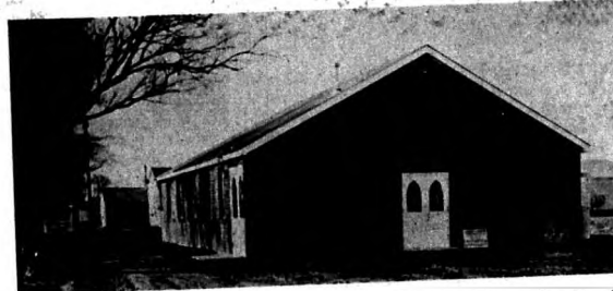
East Boundary Mission, a work sponsored by First Baptist Church, Augusta, Georgia. Cost $18,000.00 equipped.
