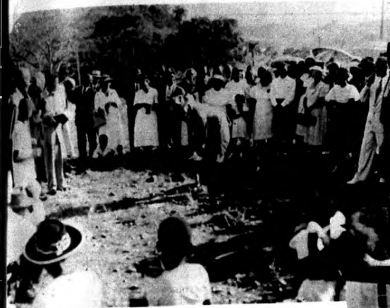
Ground-breaking service for First Baptist Church, Paraiso, Canal Zone, Rev. W. A. Walters, pastor.
