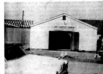
This prefabricated auditorium, first unit of the First Baptist Church, Waverly, Ohio, was put up by sixty men in one day. The second unit is now under construction.
