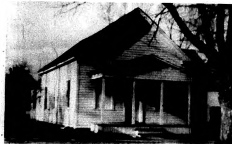
First Baptist Church, Carson City, Nevada.
