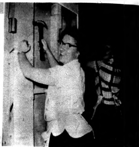
Louise Yarbrough and Helen Ruth Carpenter assist Pastor B. I. Carpenter with the building of the church at Seward, Alaska
