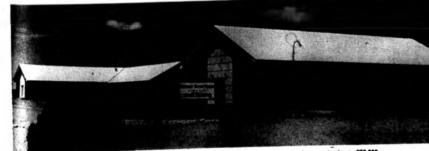
Crestview Baptist Church now has two units of a four-unit church plant. It is valued at $70,000.
