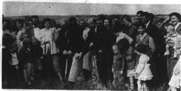
Ground-breaking services for the sanctuary were held in November, 1954. Pictured with the shovel is W. J. Fields, first convert of the church. Beside him is Pastor George Roberts, Jr.
