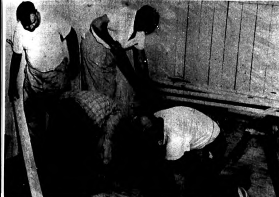
Renovation of the old depot was done by volunteer labor by the men of the church.
