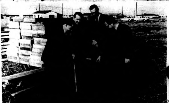
Ground breaking services for the new building of the North Richland Hills Mission of this Richland Hills Baptist Church. Rev. James Hester, mission pastor, turns the earth while Pastor Tom Lawler points out the spot. Superintendent Elton Hinz and mission committee chairman Henry McCabe smile approval.
