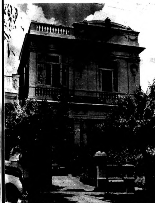
Building which inadequately houses Baptist hospital in Havana. New building critically needed.
