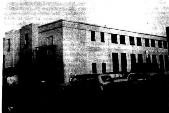
New educational plant of First Baptist Church, Anchorage, where "Mr. Baptist" (Felton Griffin) has been pastor for 12 years.
