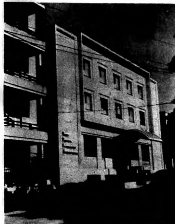
New Baptist Student Center erected during 1956 near the University of Havana campus. Dr. Ondina Maristany is in charge of the Baptist Student Union work here.
