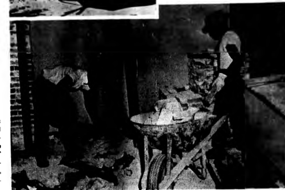
Remodeling calls for muscle and endurance. Jose Delgado of San Luis Potosi, Mexico, and Lupe Salis of Lockhart, Texas, are shown here cleaning up bricks and other debris after knocking out a wall in the old hospital building.
