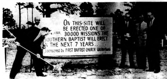
Reading left to right: Rev. W. M. Jones (breaking dirt), pastor of First Baptist Church of Walterboro, John S. Hiers, superintendent of construction, J. I. Thomas, deacon and member of missions committee, D. D. Smith, member of committee, and J. T. Givens, chairman of committee.
