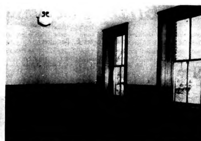
Second floor room. Repairs just completed.
