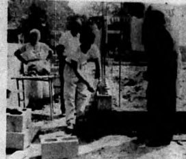
Daniel Setelo, missionary to the Spanish-speaking in El Monte, California, lays block in the construction of a new church building.
