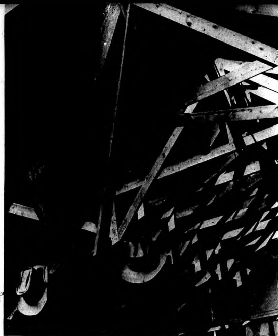
BUILDING FOR YAMPA BAPTIST CHURCH RISES AGAINST THE COLORADO SKY.
