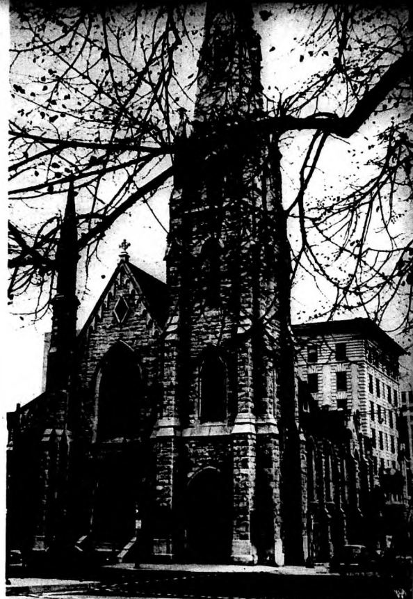
THIS PICTURESQUE CHURCH is Eutaw Place Baptist Church situated in downtown Baltimore.
