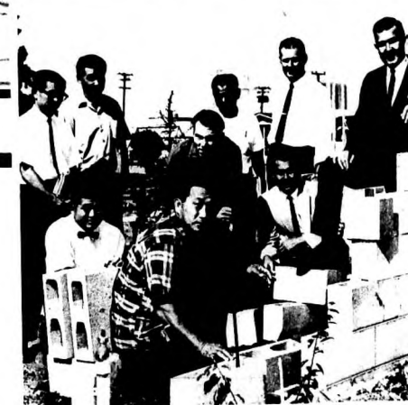
MEN OF THE CHURCH have constructed a long wall around their property as requested by the City Planning Commission.
