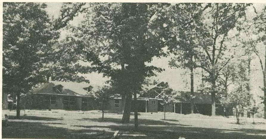
New Nursery Cottage Now Being Erected
