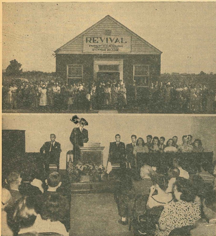
Above—New Meeting House of the Ralph Avenue Baptist Mission, east of Cane Run Road, in a fast developing area just outside the city limits of Louisville. The dozen charter members are shown on the right standing with J. Perry Carter, Superintendent of City Missions.
