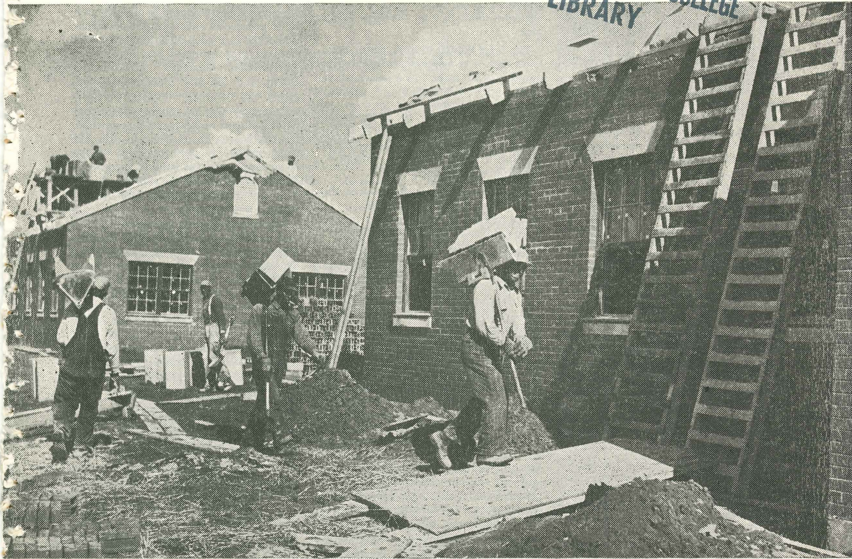
The New Spring Meadows Begins to Take Shape at Middletown, Kentucky (See Story on Page 9)
