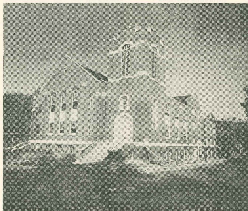
New Auditorium and Educational Plant of the First Baptist Church of Harlan, Ky.
