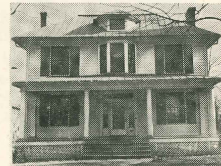
The Beechmont Annex
